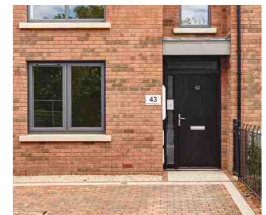
Painted timber doors at own door ground floor apartments
