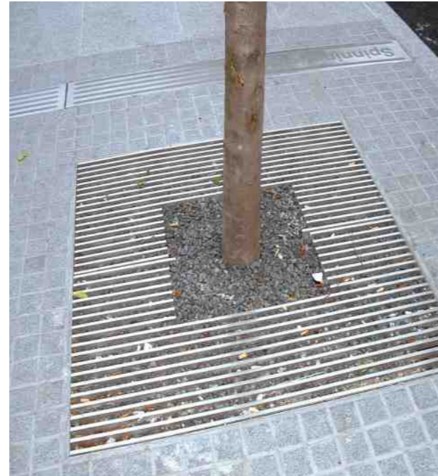
Landscape details in public realm - tree grilles on Market Street and permeable paving at on-street parking bays
