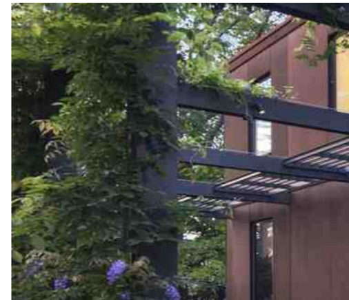
Painted steel pergola structure
