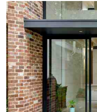
Powder coated aluminium doors and prefinished metal canopy to residential entrance cores
