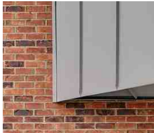
Profiled zinc or similar cladding
